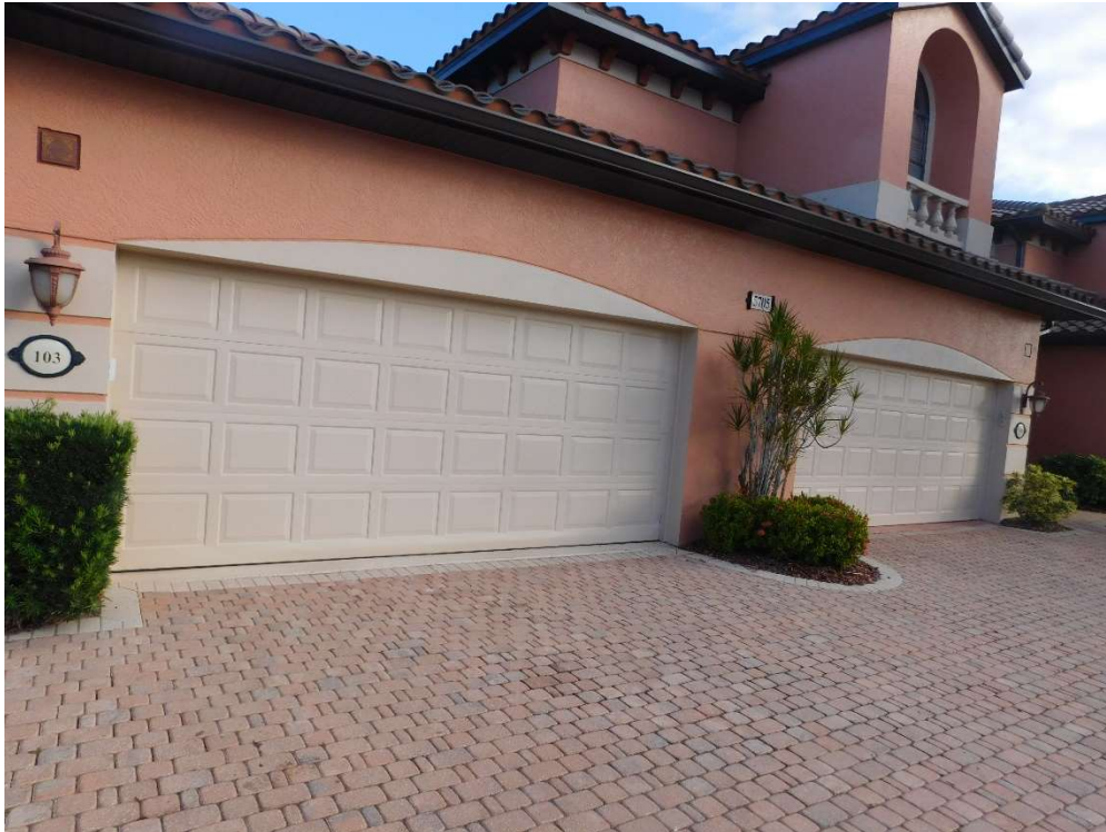
View of non-glazed openings (per question 7).
