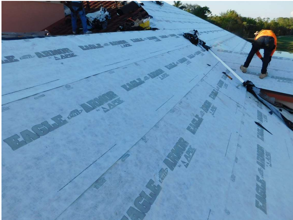
View of self-adhering roofing underlayment (per question 6).
