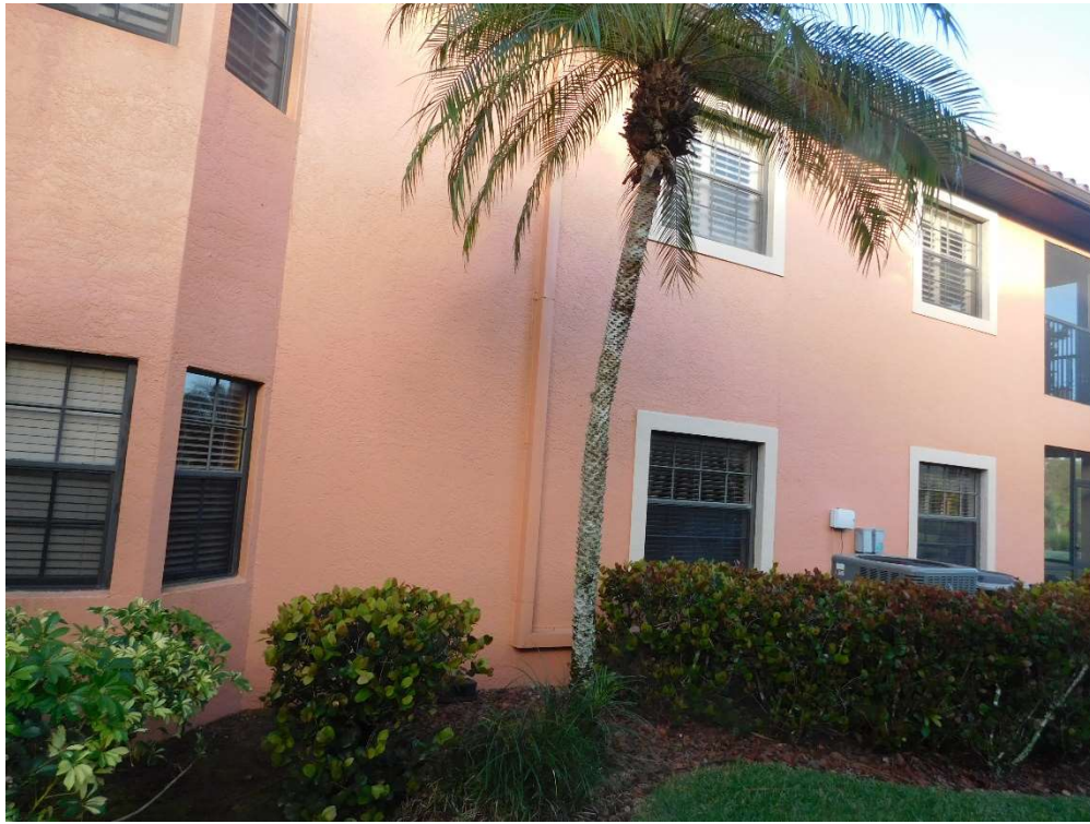
View of typical glazed openings (per question 7).
