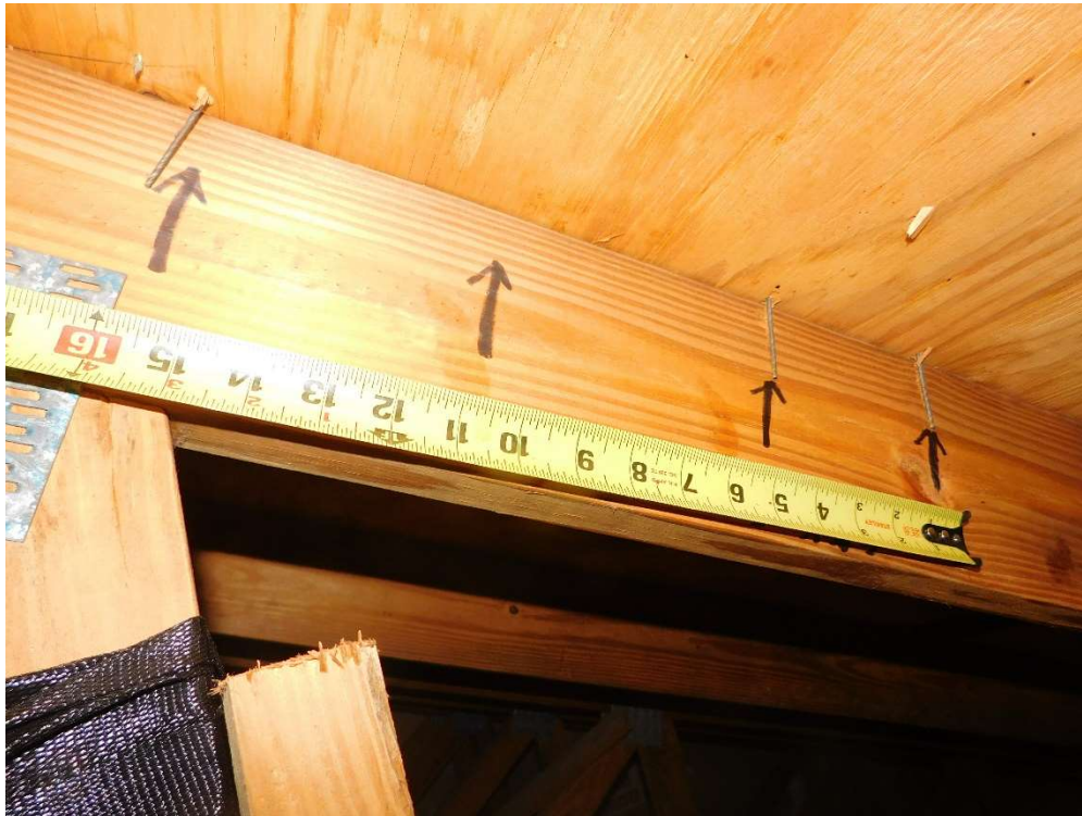
View of re-nailing pattern (per question 3).
