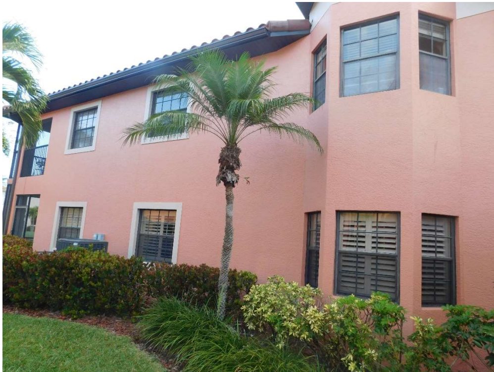
View of typical glazed openings (per question 7).
