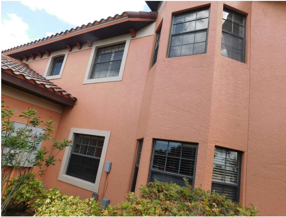
View of typical glazed openings (per question 7).
