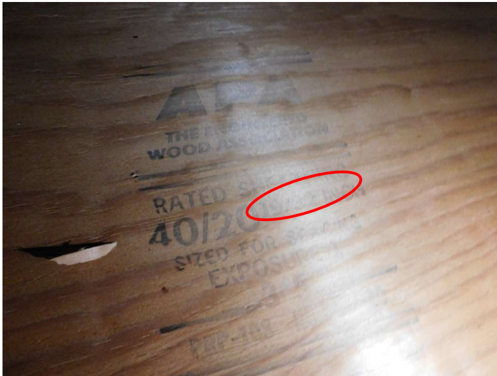
View of existing plywood sheathing thickness (19/32) per question 3.
