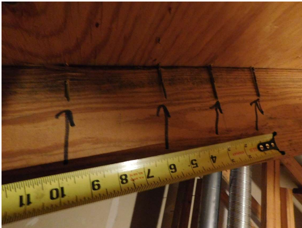
View of re-nailing pattern (per question 3).
