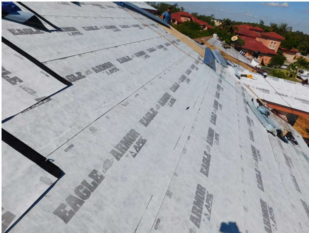
View of self-adhering roofing underlayment (per question 6).
