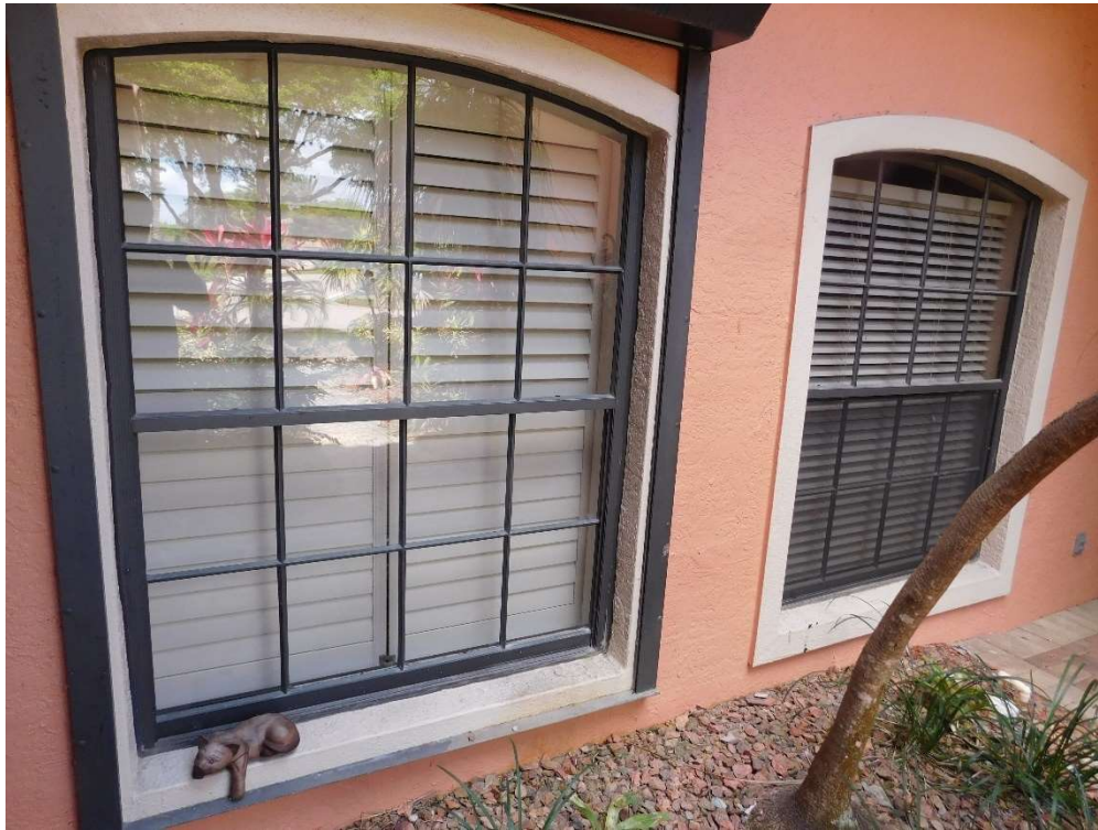
View of typical glazed openings (per question 7).
