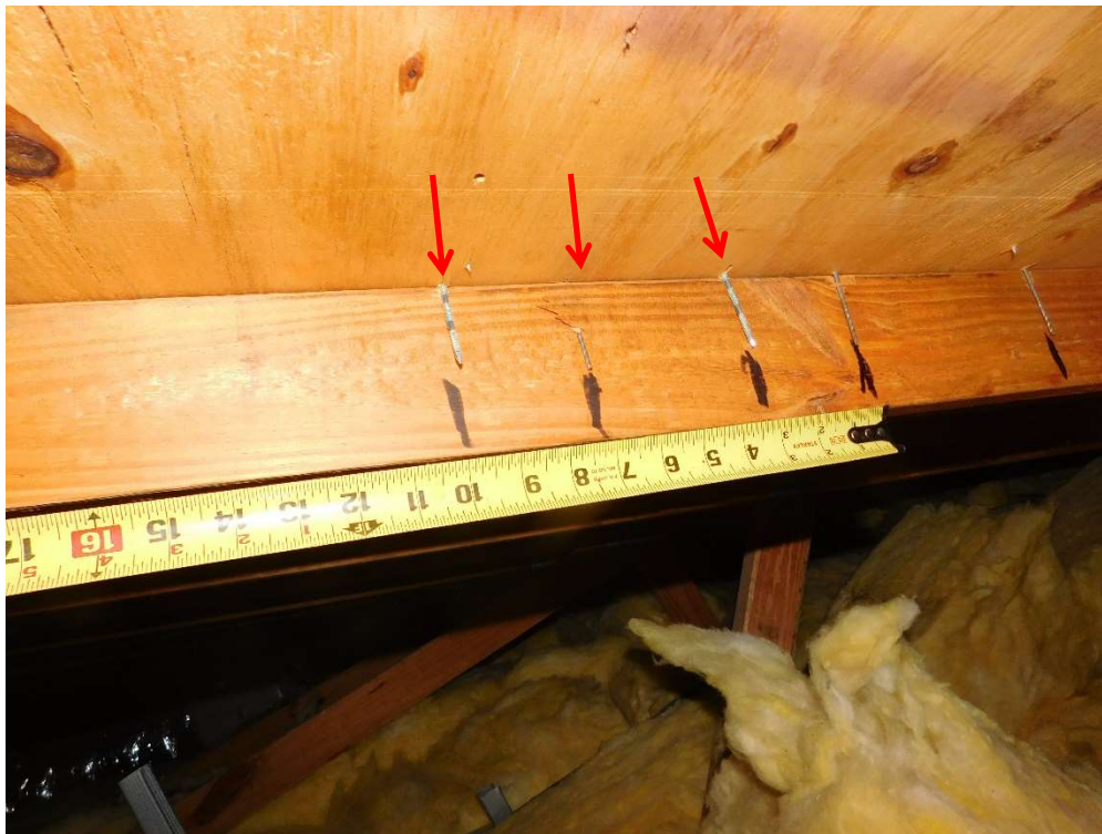
View of re-nailing pattern (per question 3).
