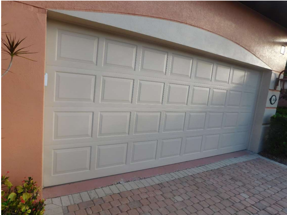
View of non-glazed openings (per question 7).
