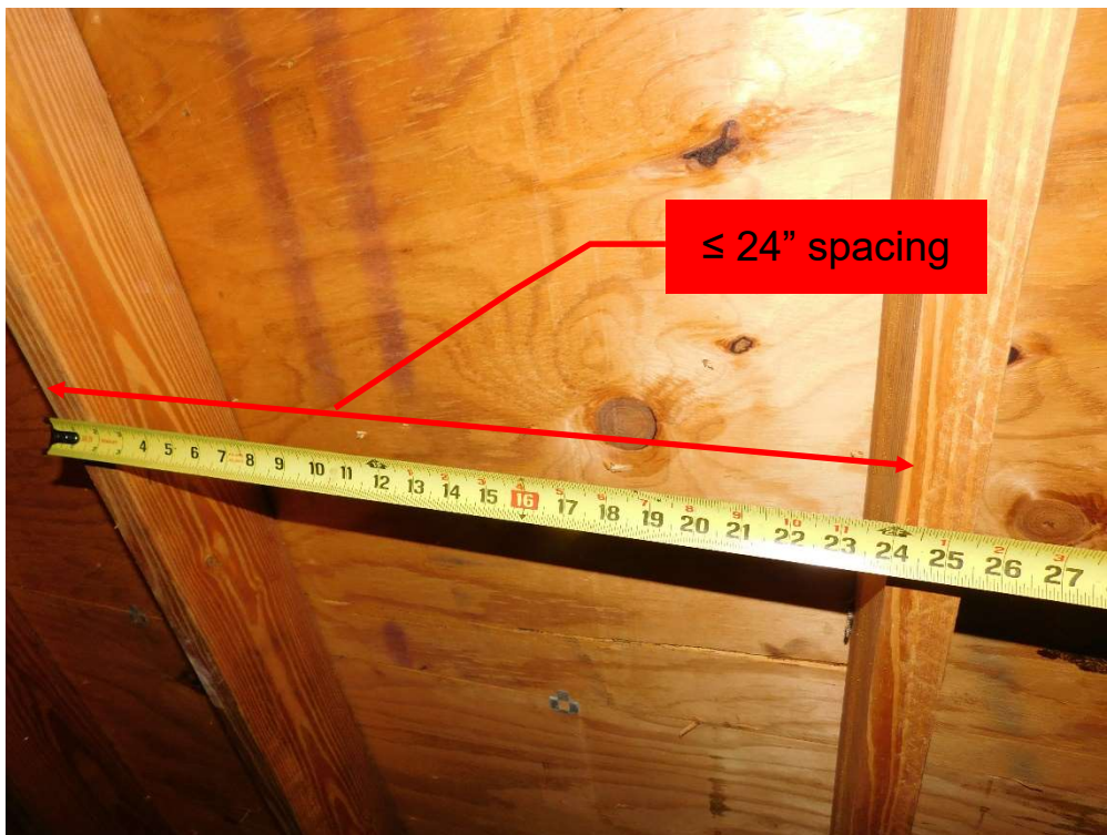
View of truss spacing (per question 3).
