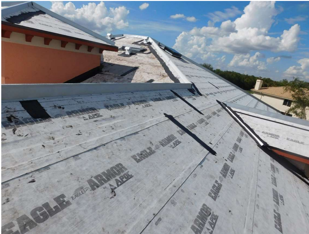
View of self-adhering roofing underlayment (per question 6).
