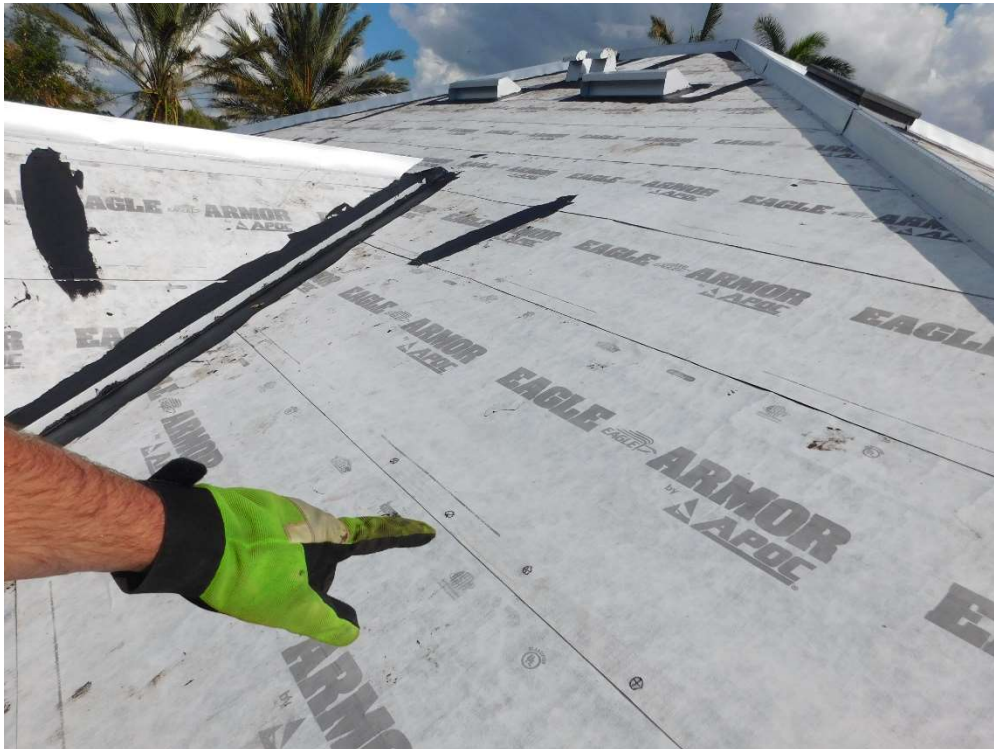
View of self-adhering roofing underlayment (per question 6).
