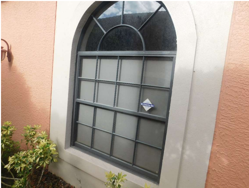
View of typical glazed openings (per question 7).
