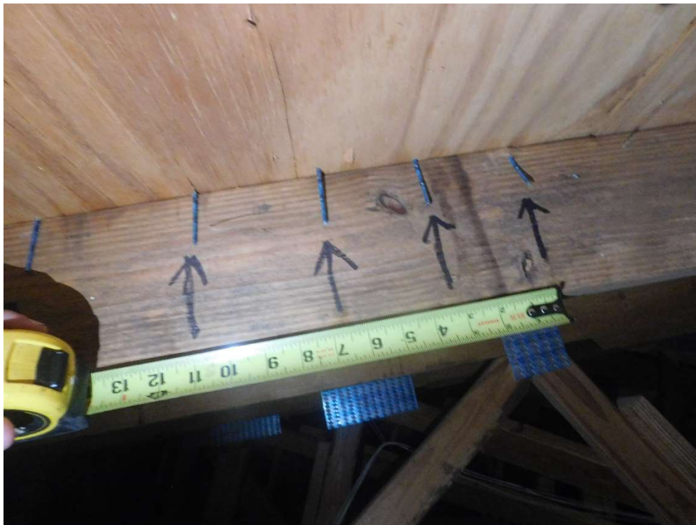
View of re-nailing pattern (per question 3).
