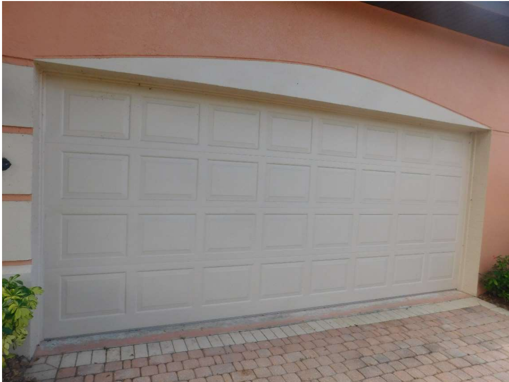
View of non-glazed openings (per question 7).
