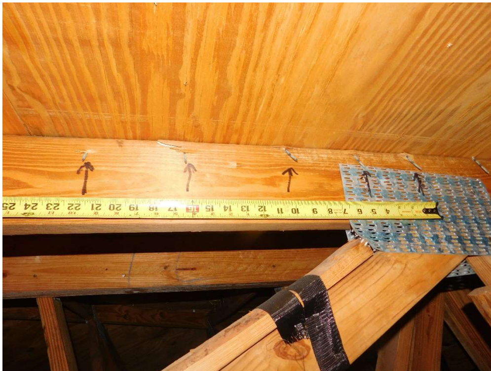
View of re-nailing pattern (per question 3).
