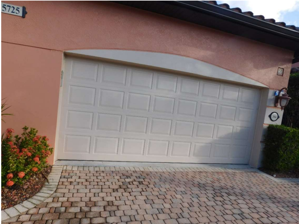
View of non-glazed openings (per question 7).
