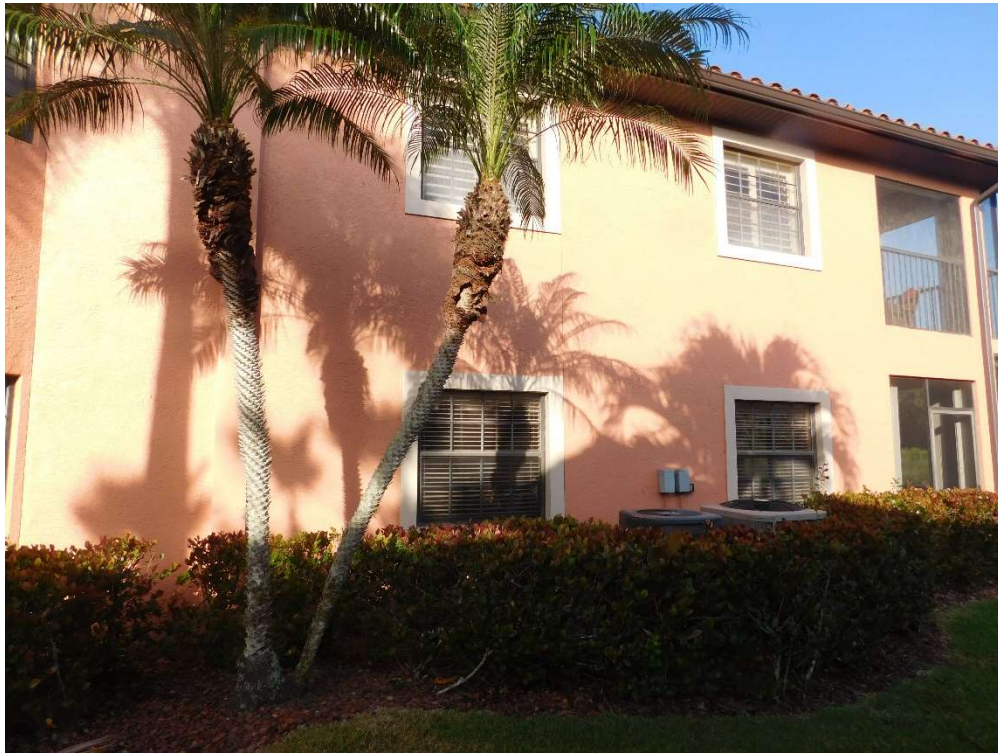
View of typical glazed openings (per question 7).
