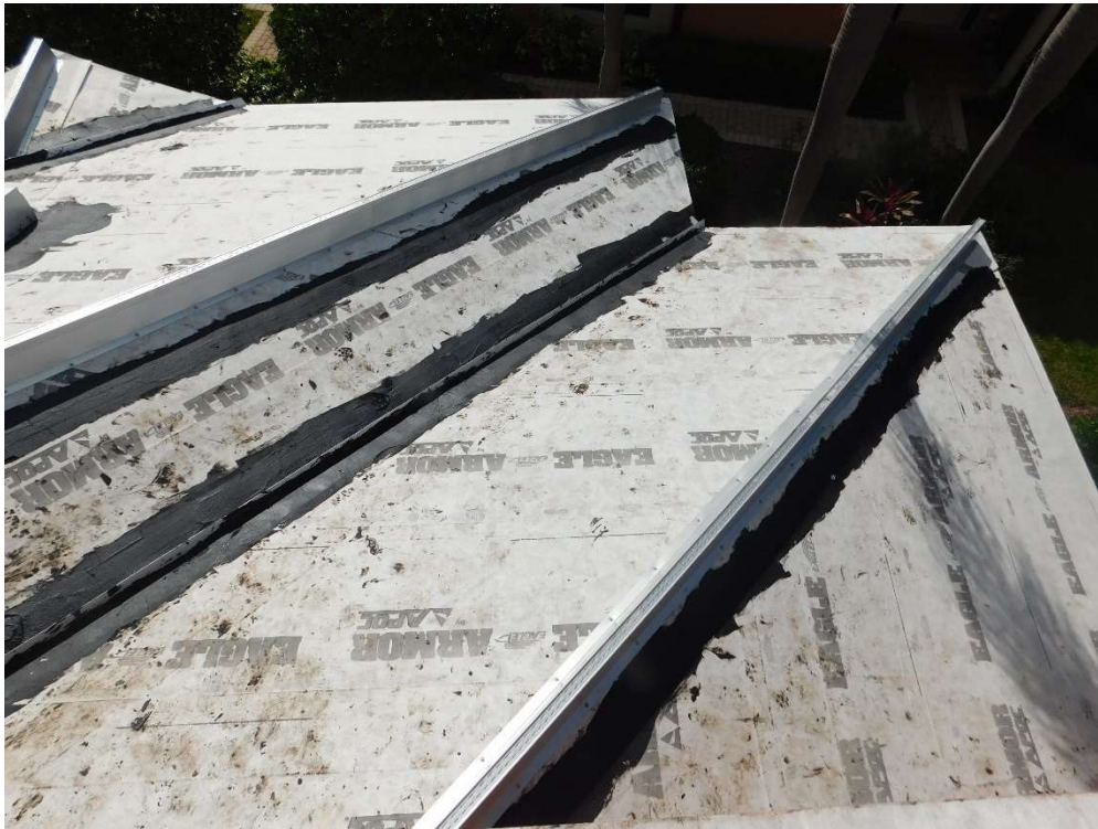
View of self-adhering roofing underlayment (per question 6).
