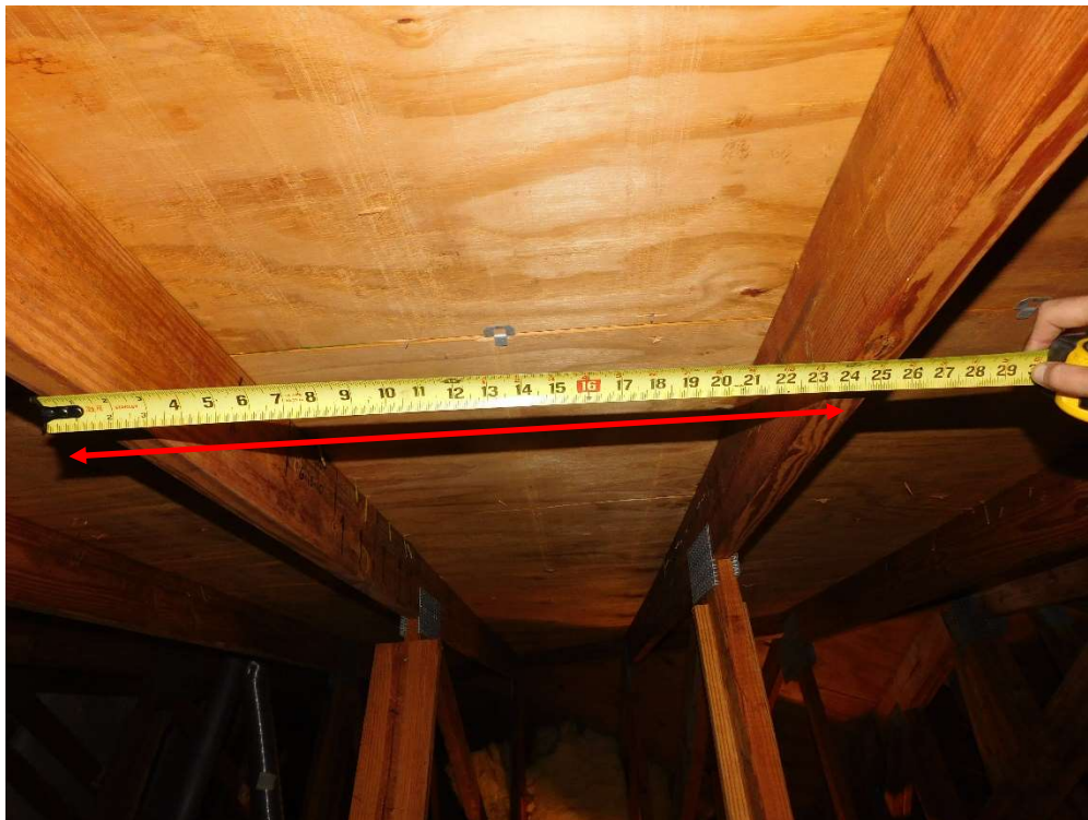
View of truss spacing (per question 3).
