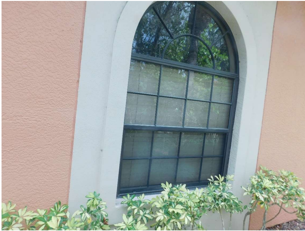
View of typical glazed openings (per question 7).
