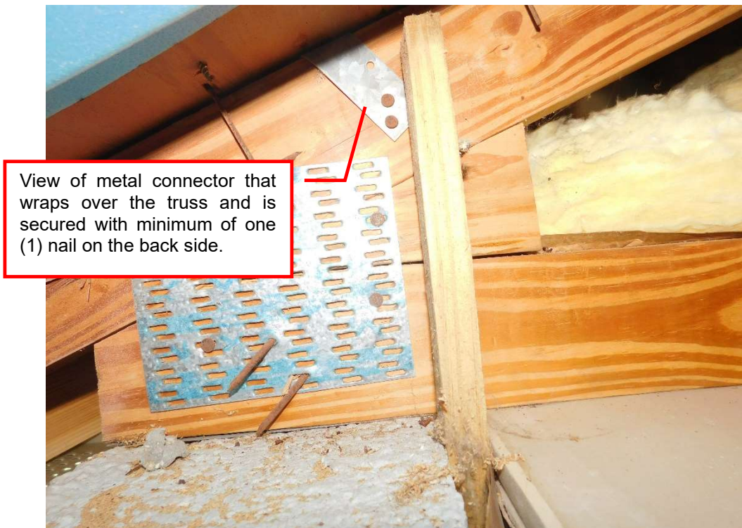
View of metal connector used on Roof to Wall attachment (per question 4).
