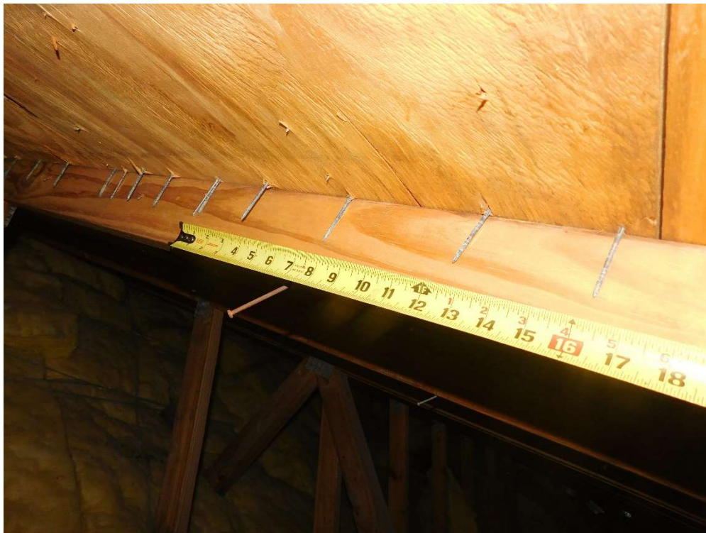
View of re-nailing pattern (per question 3).
