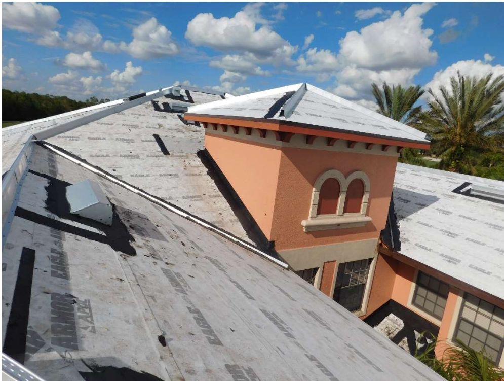
View of self-adhering roofing underlayment (per question 6).
