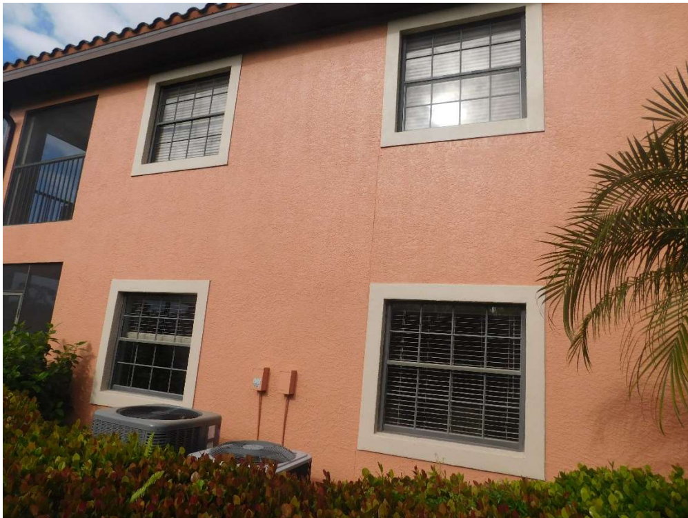
View of typical glazed openings (per question 7).
