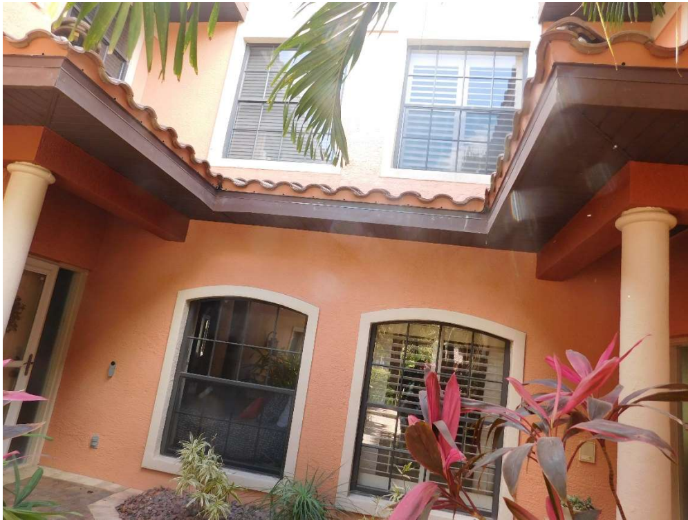
View of typical glazed openings (per question 7).
