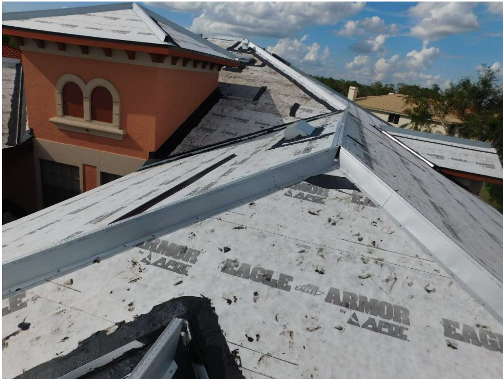
View of self-adhering roofing underlayment (per question 6).
