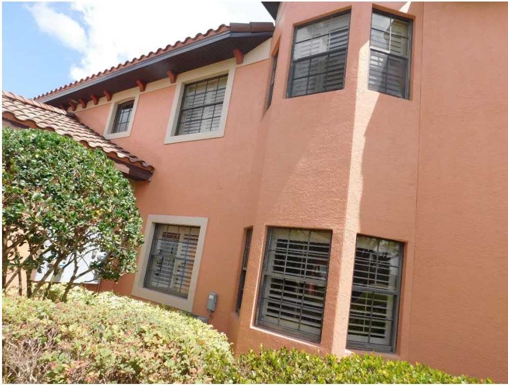
View of typical glazed openings (per question 7).
