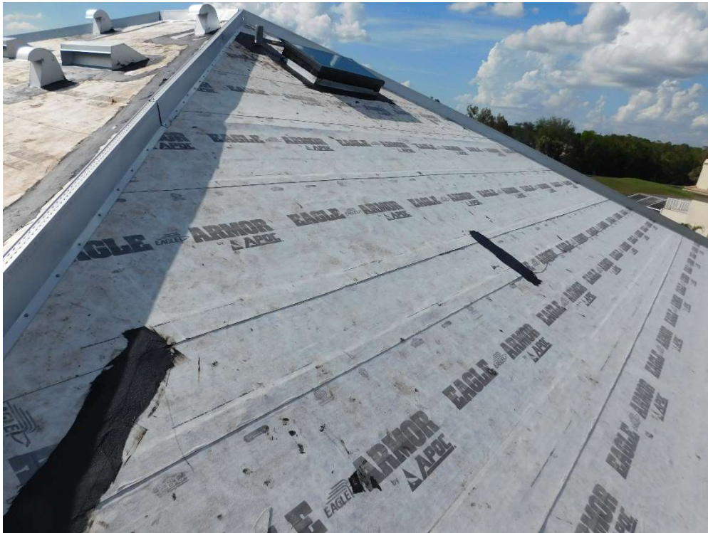
View of self-adhering roofing underlayment (per question 6).
