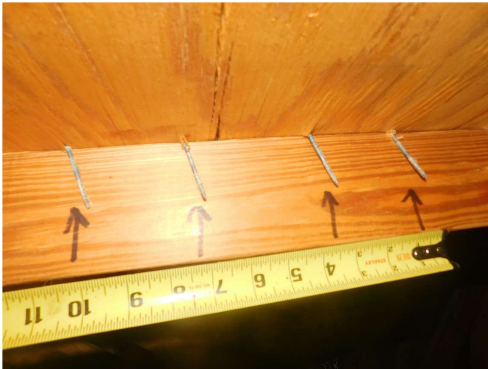
View of re-nailing pattern (per question 3).
