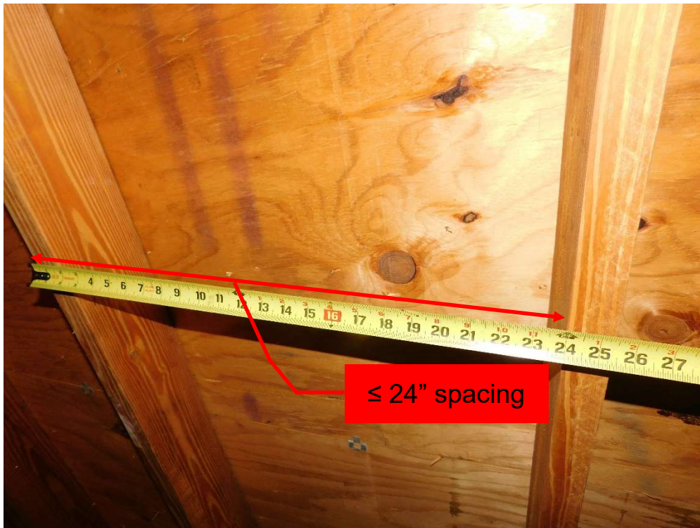
View of truss spacing (per question 3).
