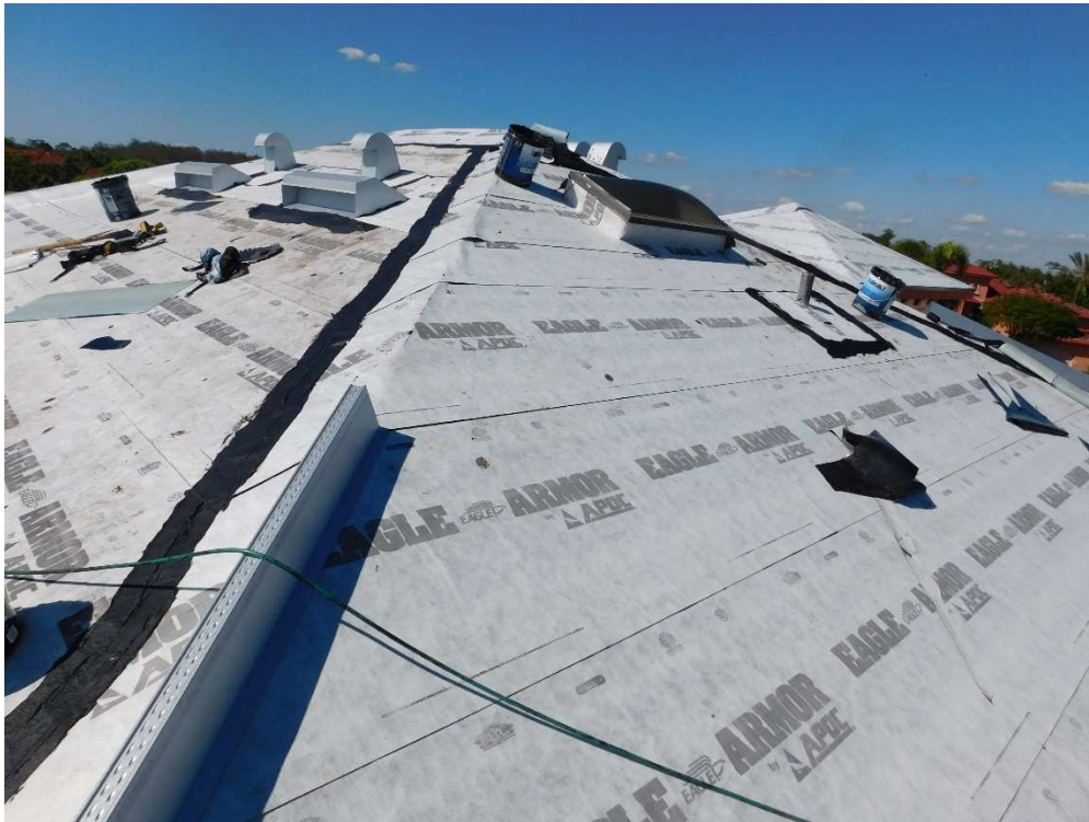
View of self-adhering roofing underlayment (per question 6).
