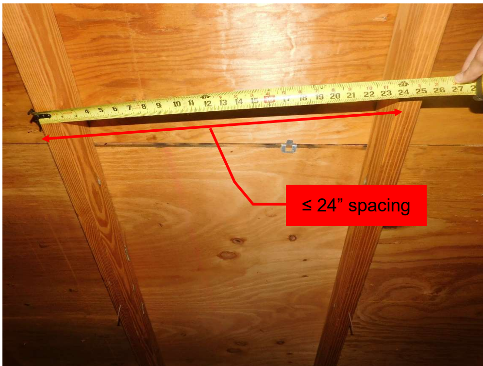
View of truss spacing (per question 3).
