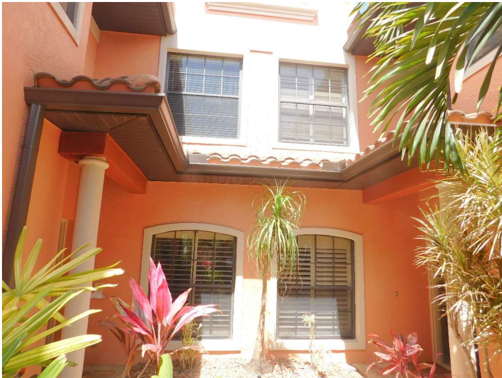
View of typical glazed openings (per question 7).
