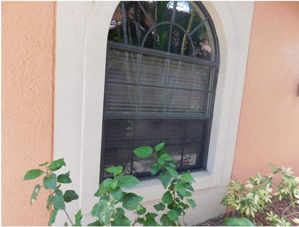
View of typical glazed openings (per question 7).
