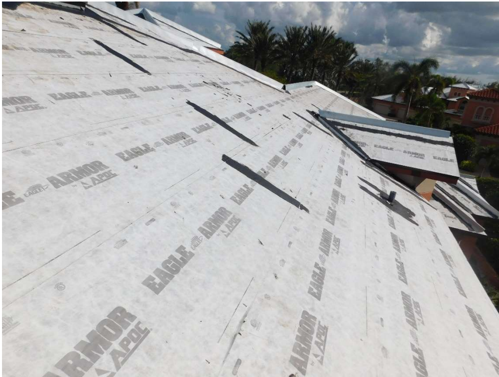
View of self-adhering roofing underlayment (per question 6).
