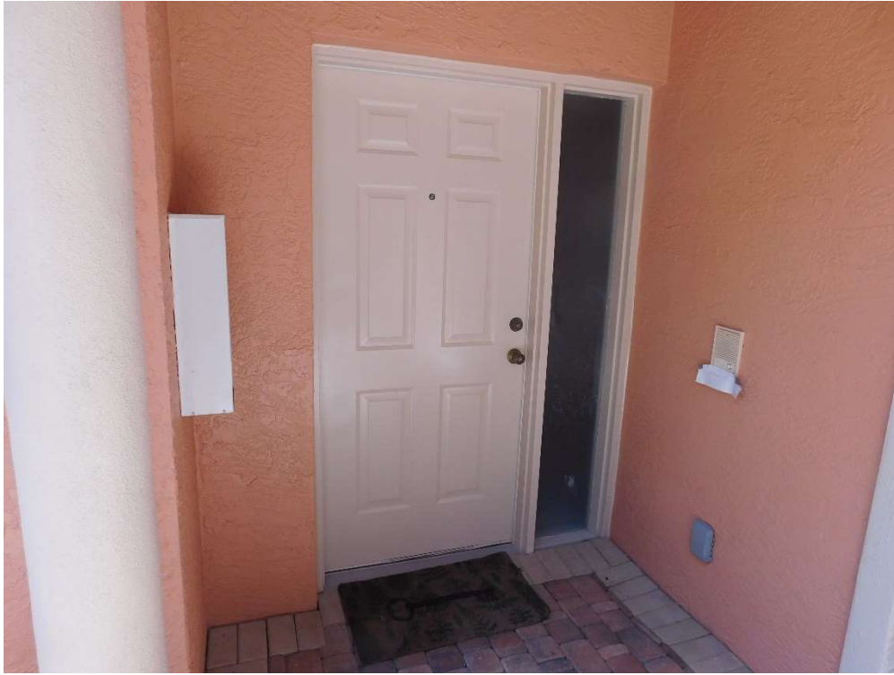
View of typical glazed openings (per question 7).
