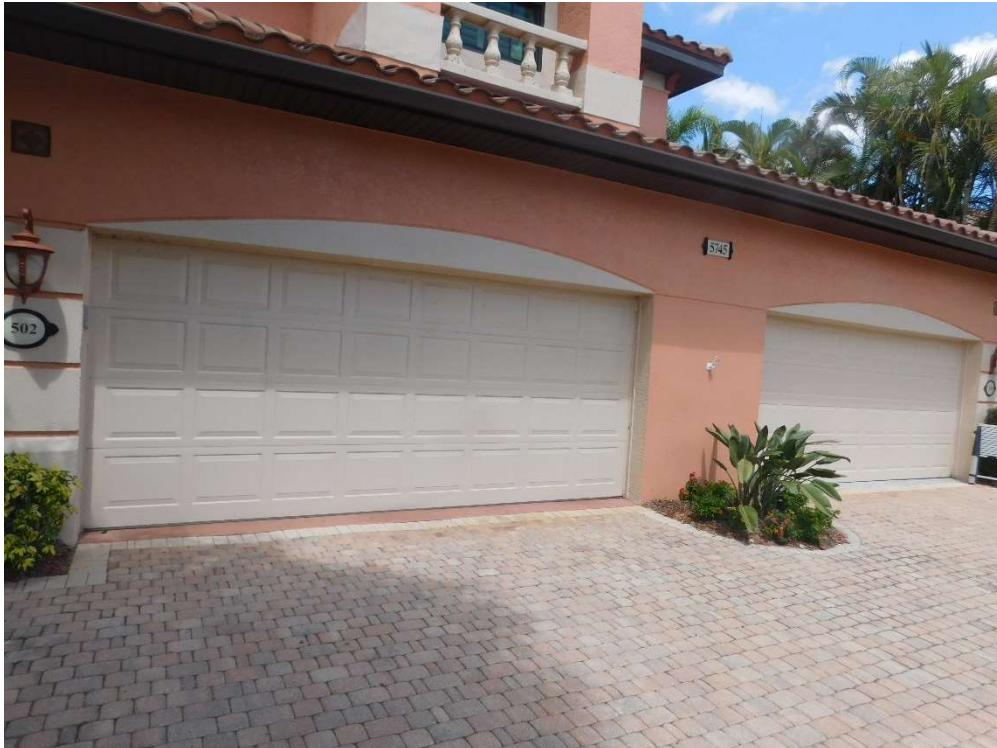
View of unglazed openings (per question 7).
