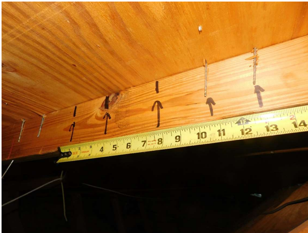
View of re-nailing pattern (per question 3).
