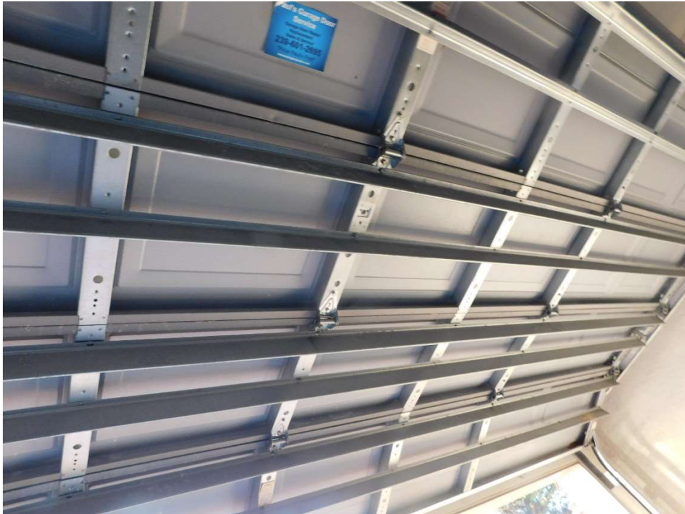
View of non-glazed openings (per question 7).
