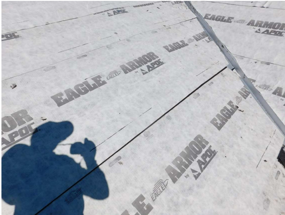
View of self-adhering roofing underlayment (per question 6).
