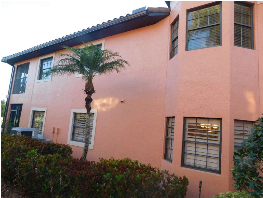
View of typical glazed openings (per question 7).
