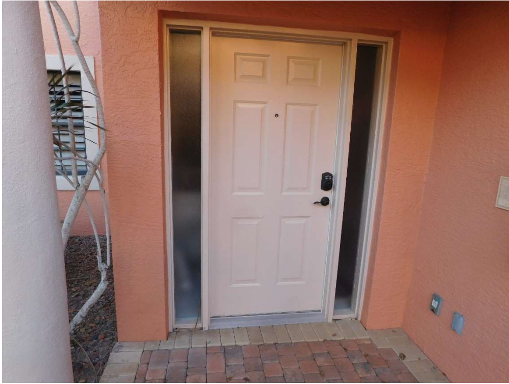
View of typical glazed openings (per question 7).
