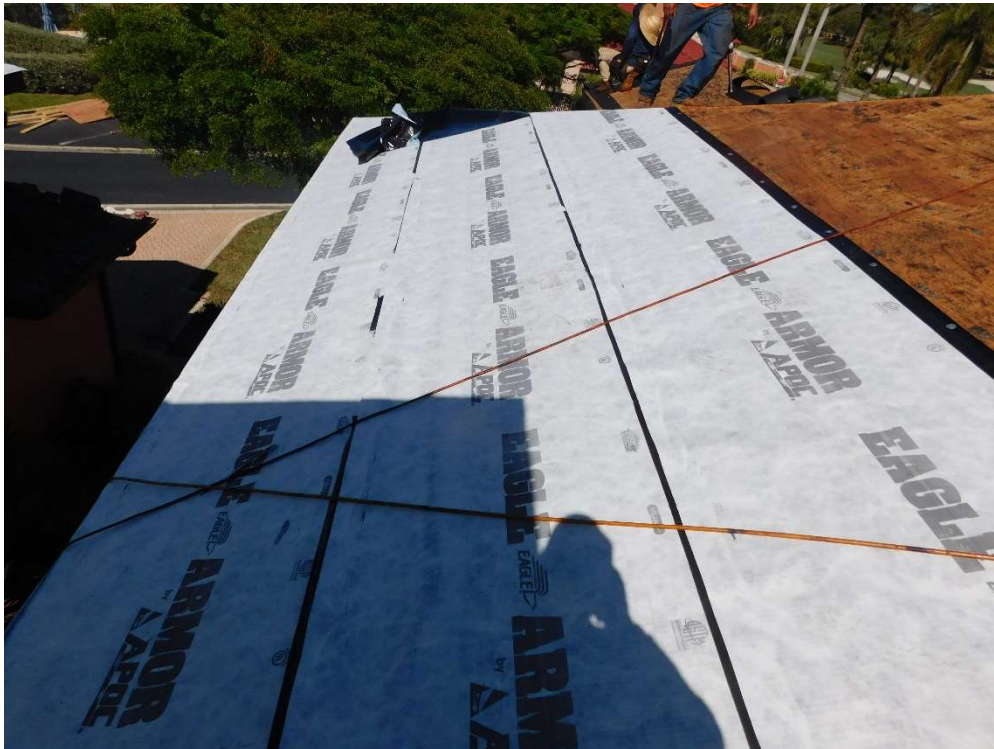
View of self-adhering roofing underlayment (per question 6).
