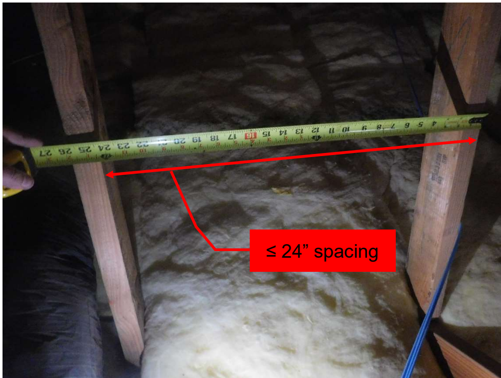
View of truss spacing (per question 3).
