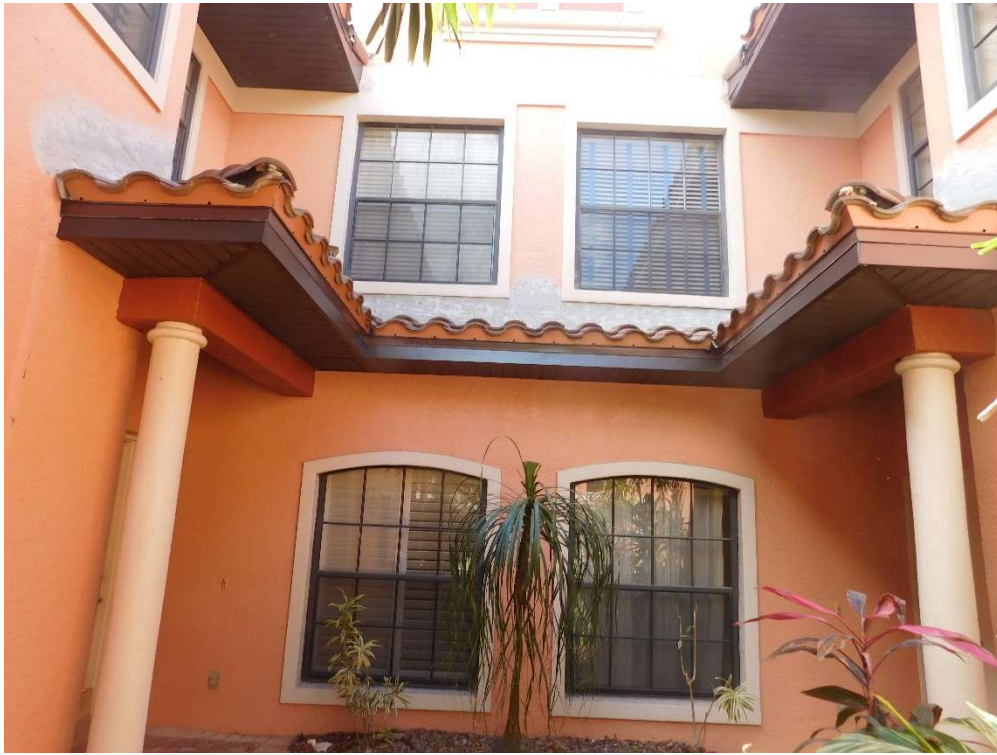
View of typical glazed openings (per question 7).
