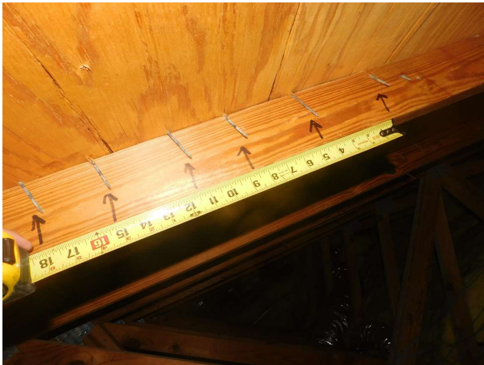
View of re-nailing pattern (per question 3).
