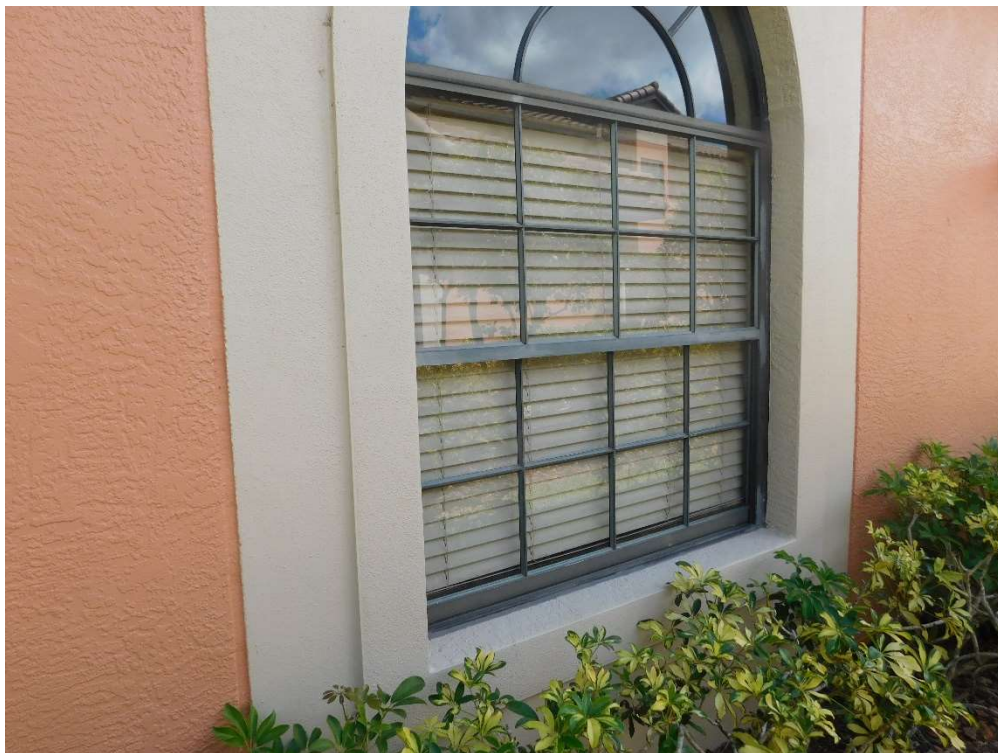
View of typical glazed openings (per question 7).
