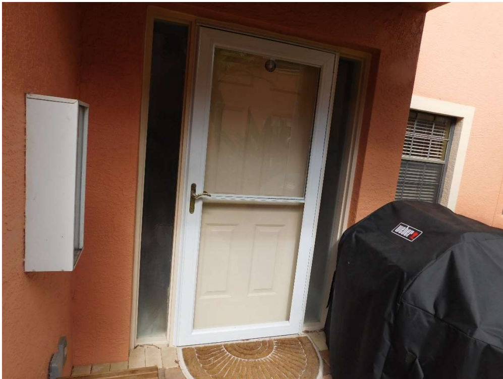
View of typical glazed openings (per question 7).
