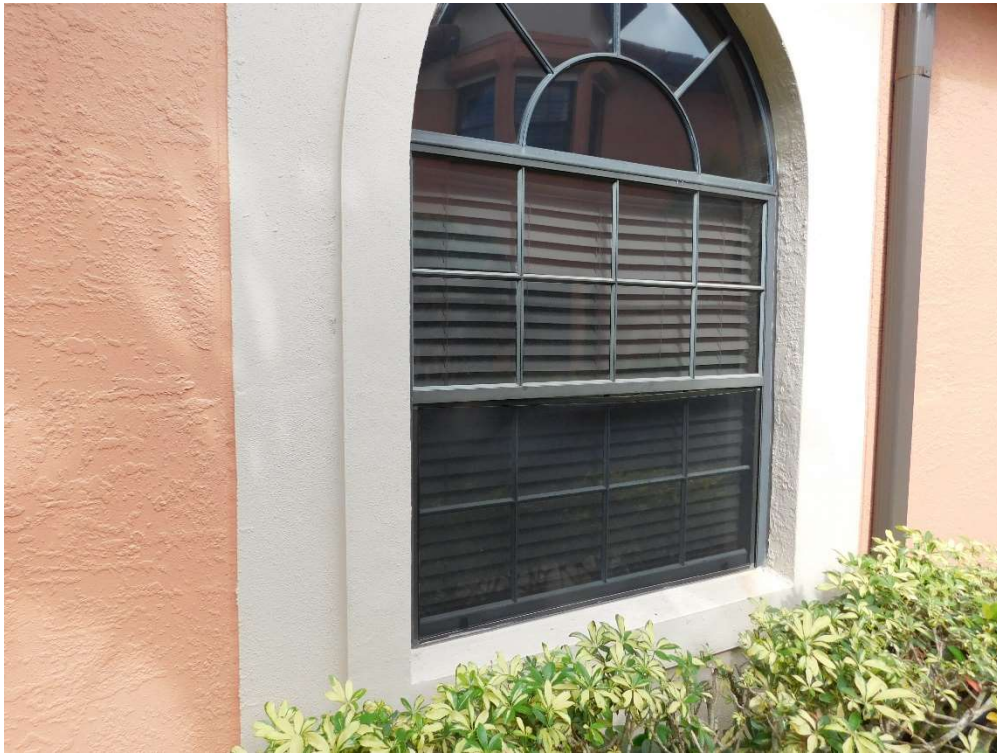
View of typical glazed openings (per question 7).
