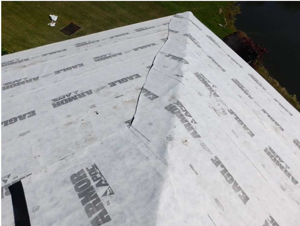
View of self-adhering roofing underlayment (per question 6).
