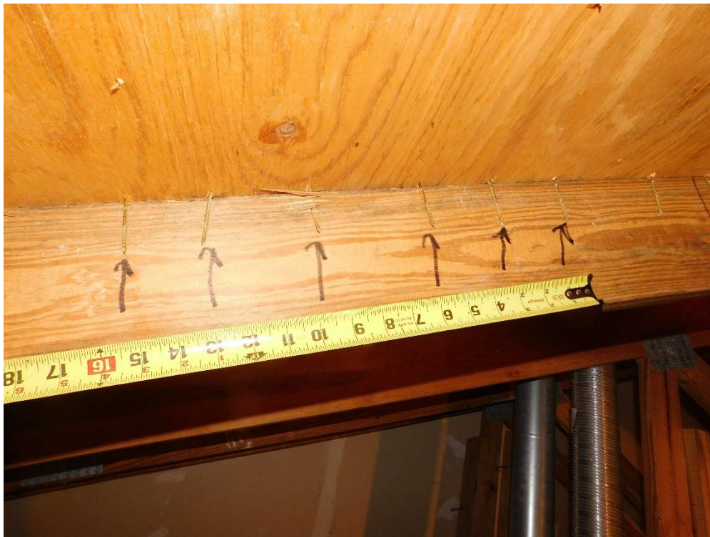
View of re-nailing pattern (per question 3).
