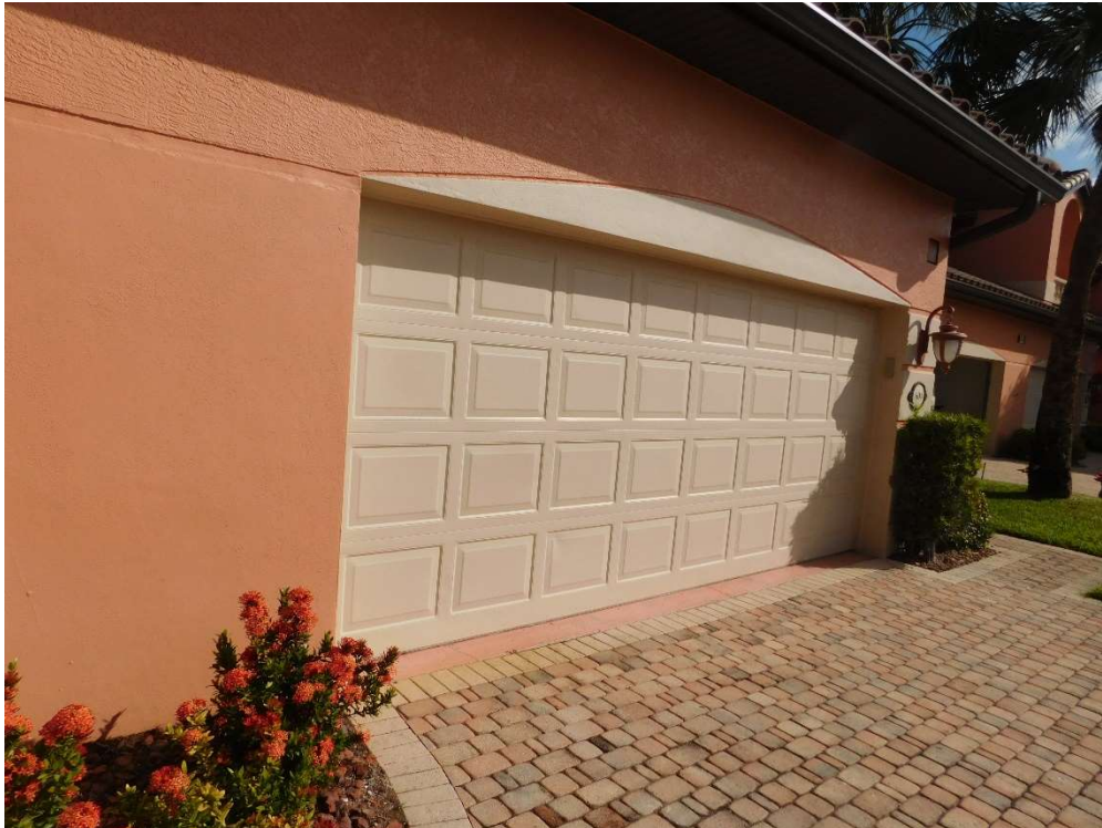
View of non-glazed openings (per question 7).
