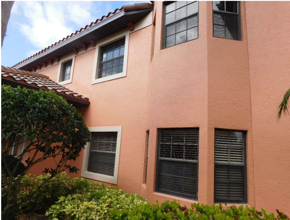
View of typical glazed openings (per question 7).
