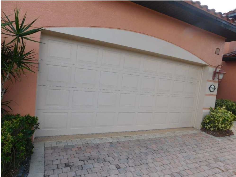
View of typical unglazed openings (per question 7).
