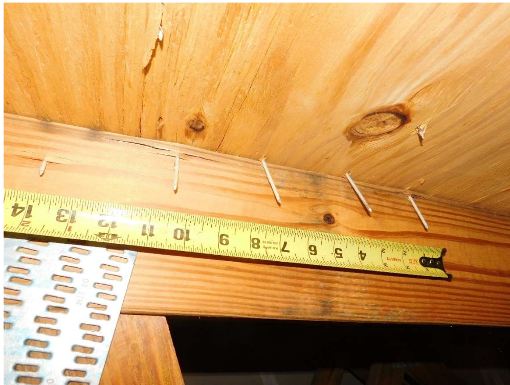
View of re-nailing pattern (per question 3).
