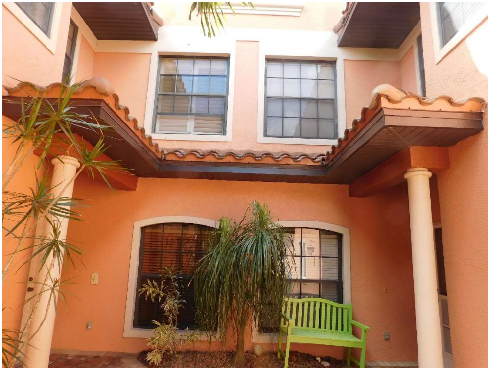
View of typical glazed openings (per question 7).
