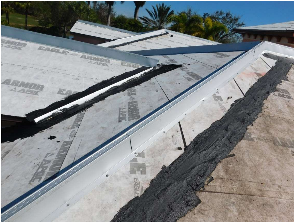
View of self-adhering roofing underlayment (per question 6).
