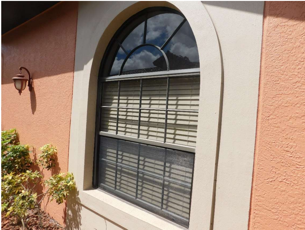
View of typical glazed openings (per question 7).
