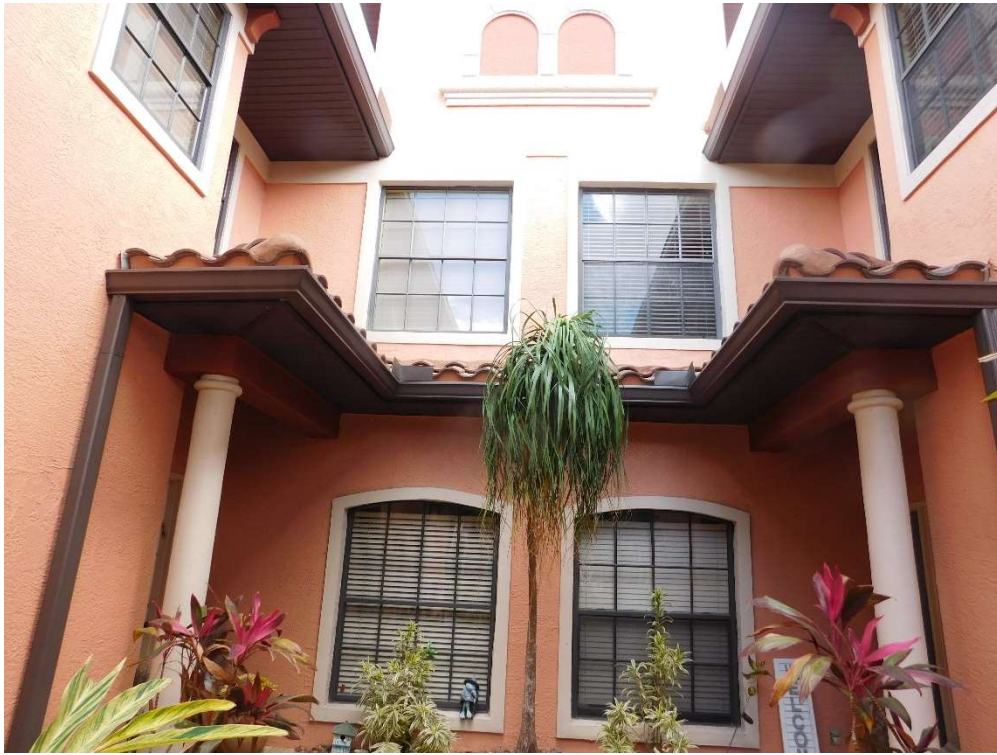
View of typical glazed openings (per question 7).
