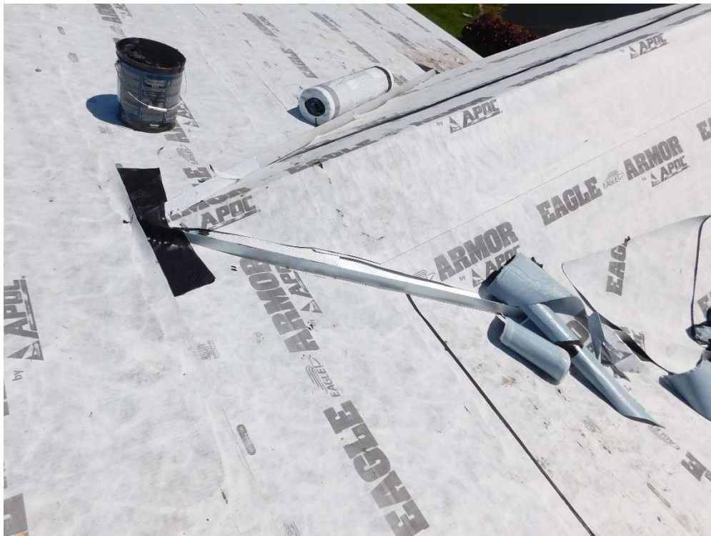
View of self-adhering roofing underlayment (per question 6).
