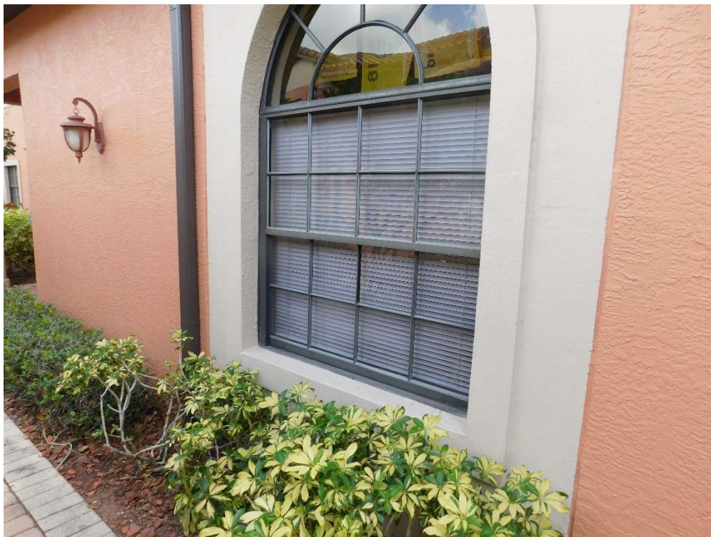
View of typical glazed openings (per question 7).
