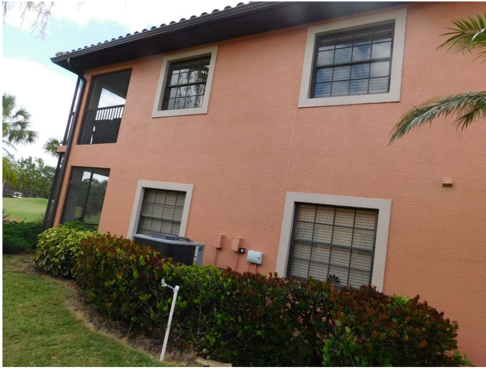
View of typical glazed openings (per question 7).
