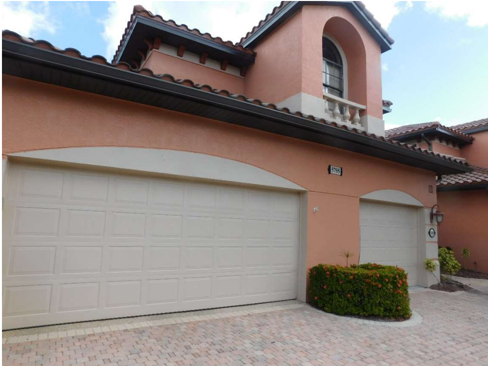
View of non-glazed openings (per question 7).
