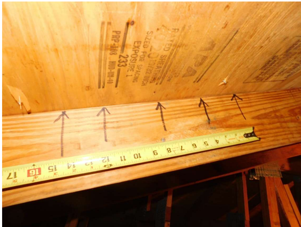
View of re-nailing pattern (per question 3).
