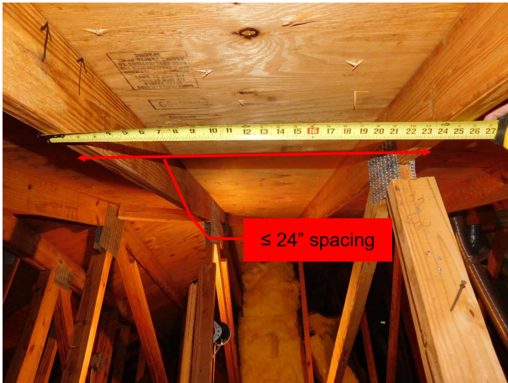
View of truss spacing (per question 3).
