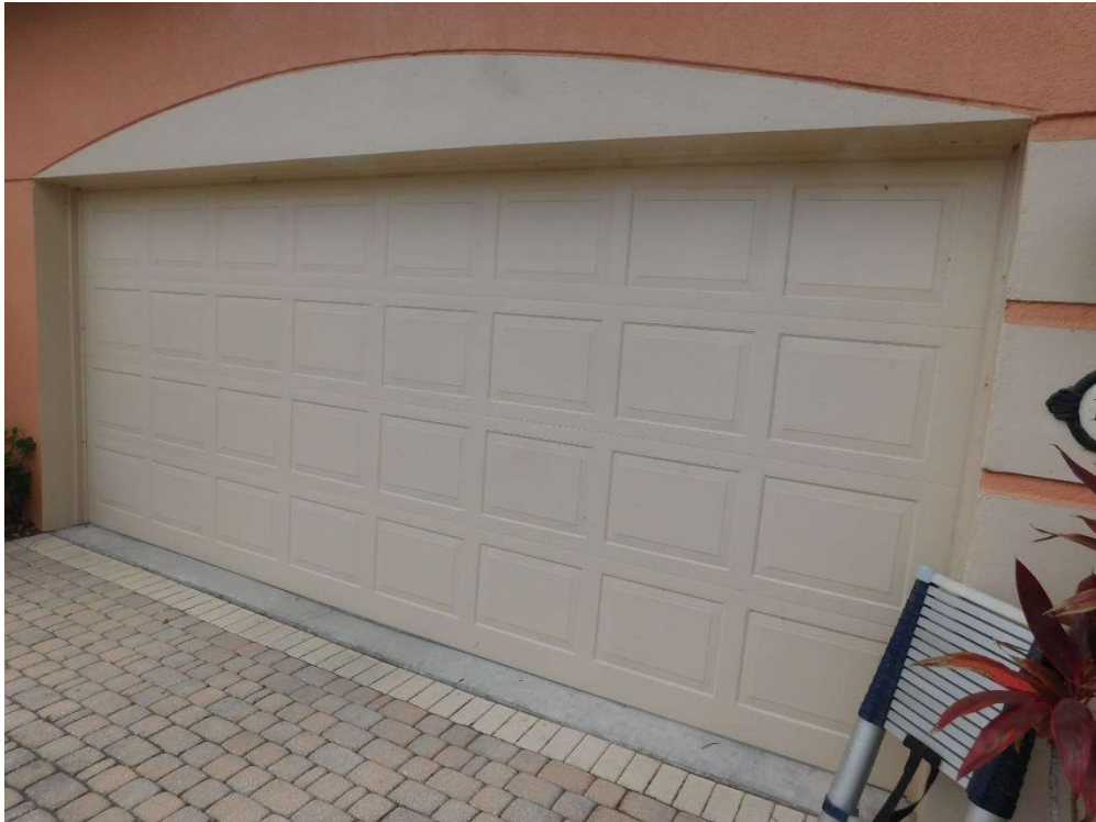
View of non-glazed openings (per question 7).
