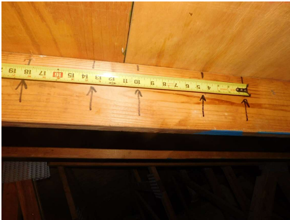
View of re-nailing pattern (per question 3).
