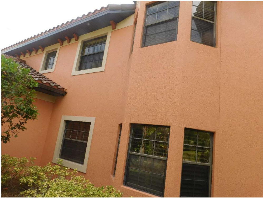
View of typical glazed openings (per question 7).
