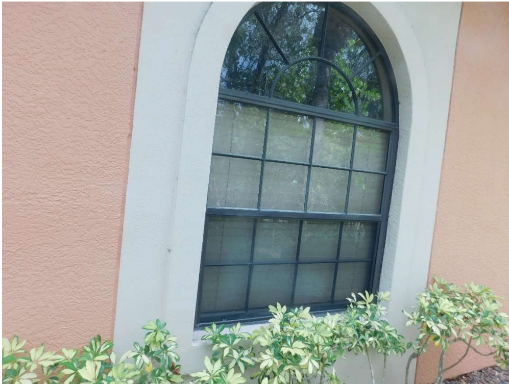
View of typical glazed openings (per question 7).
