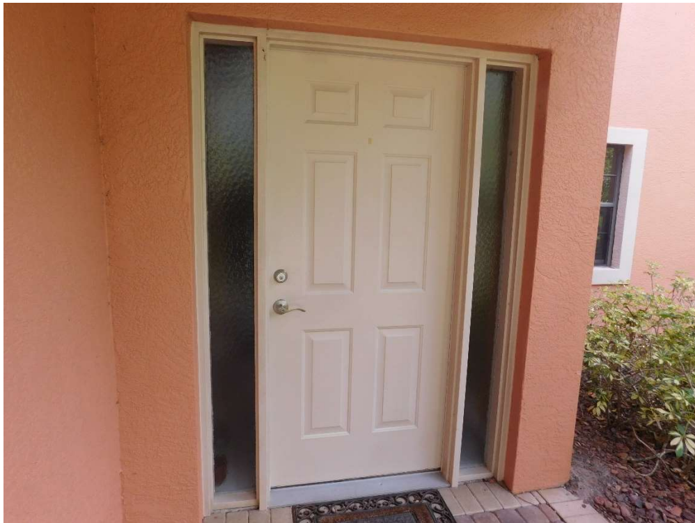
View of typical glazed openings (per question 7).
