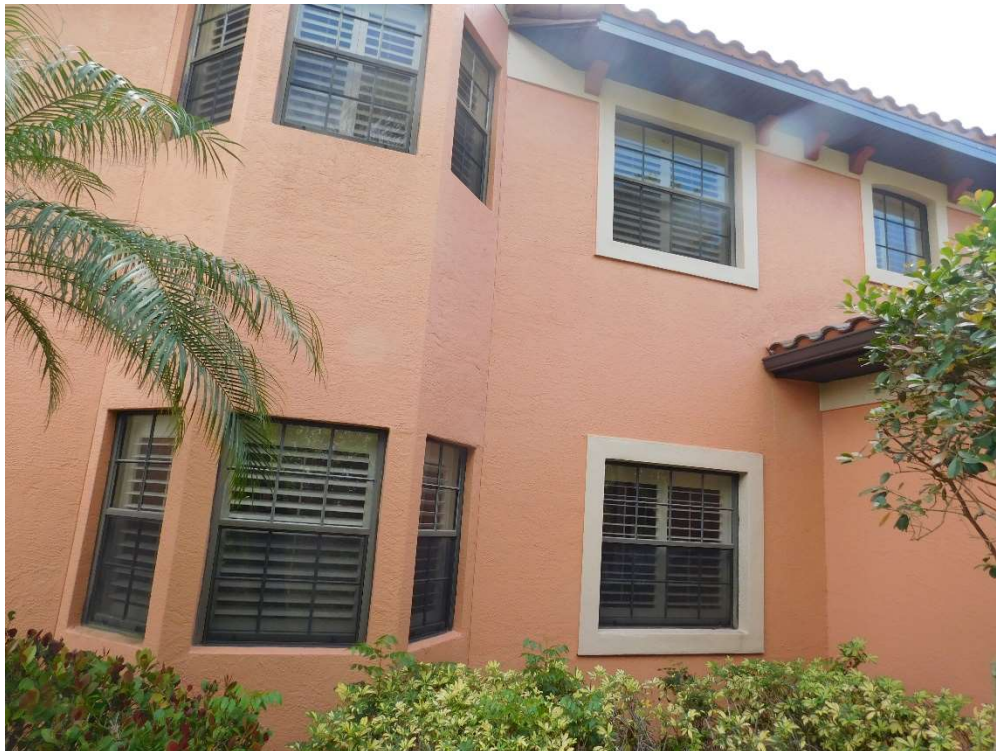
View of typical glazed openings (per question 7).
