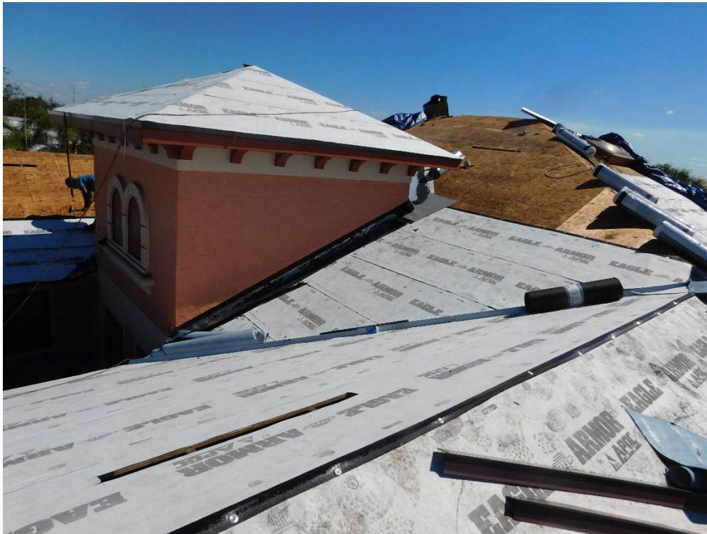
View of self-adhering roofing underlayment (per question 6).
