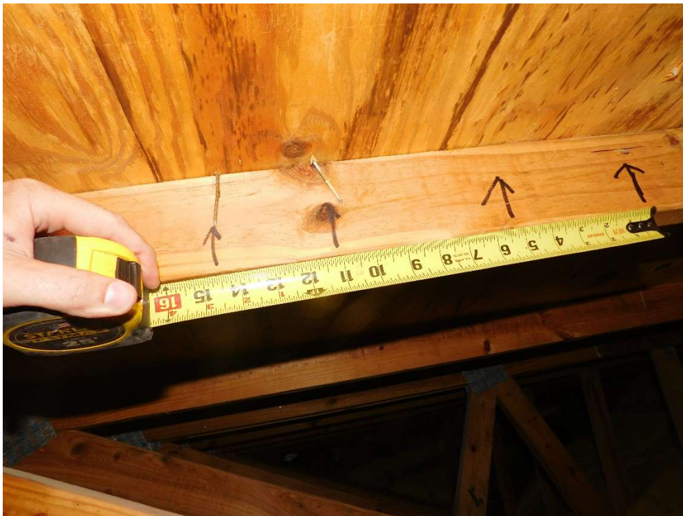
View of re-nailing pattern (per question 3).
