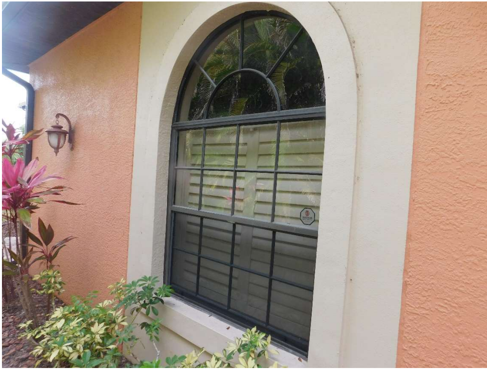
View of typical glazed openings (per question 7).
