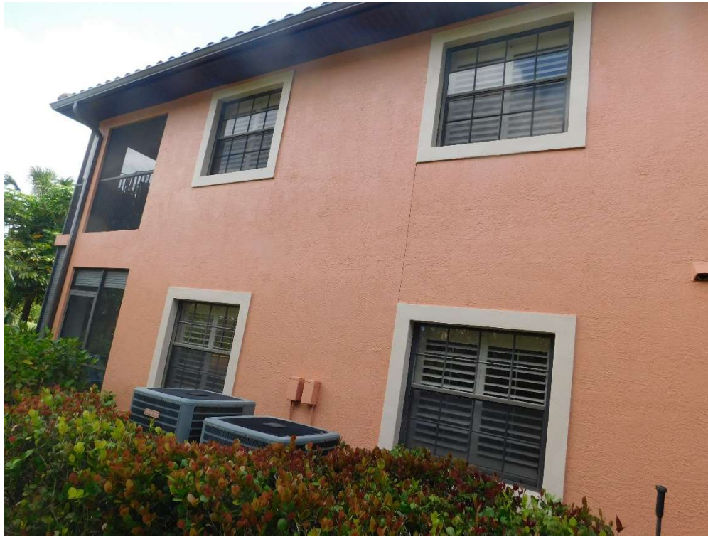
View of typical glazed openings (per question 7).
