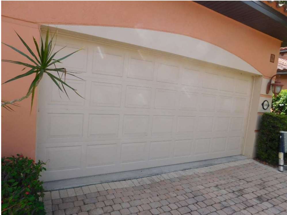
View of non-glazed openings (per question 7).
